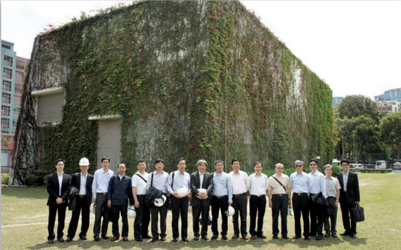
A delegation from the Ningbo Municipal Flood Control and Drought Relief Office visited the Tai Hang Tung Underground Storm water Storage Tank in March 2013
